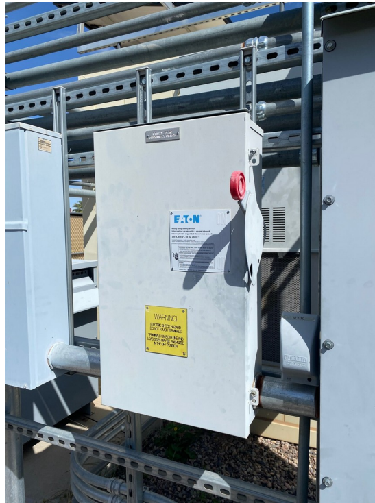
Figure A-4 - Enclosed utility disconnect example
