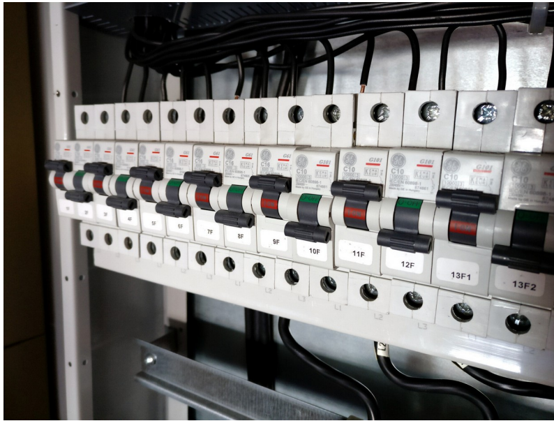
Figure A-11 - DIN-rail miniature circuit breakers
