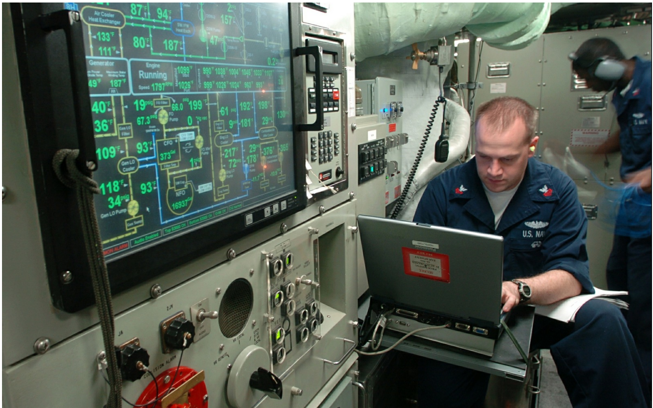
Figure 11-4 - Diesel generator control panel
