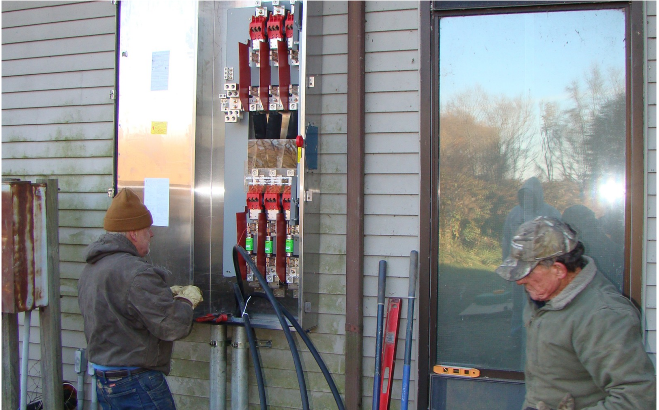
Figure 11-3 - Backup-generator junction-panel installation
