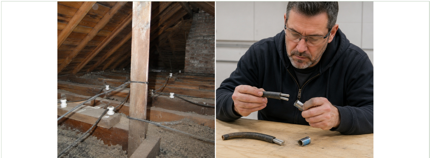
Left: knob-and-tube wiring. Right: disconnected aluminum cable being checked.
