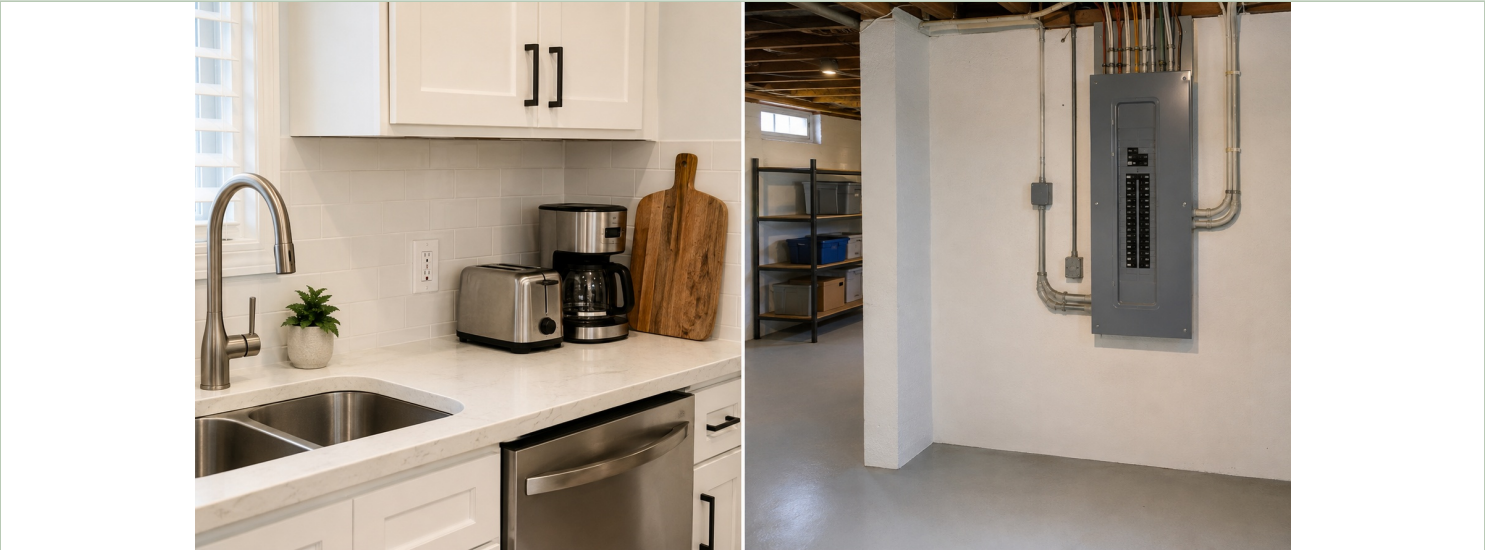
Left: kitchen receptacle and appliances. Right: clear, dry access to a closed panel.
