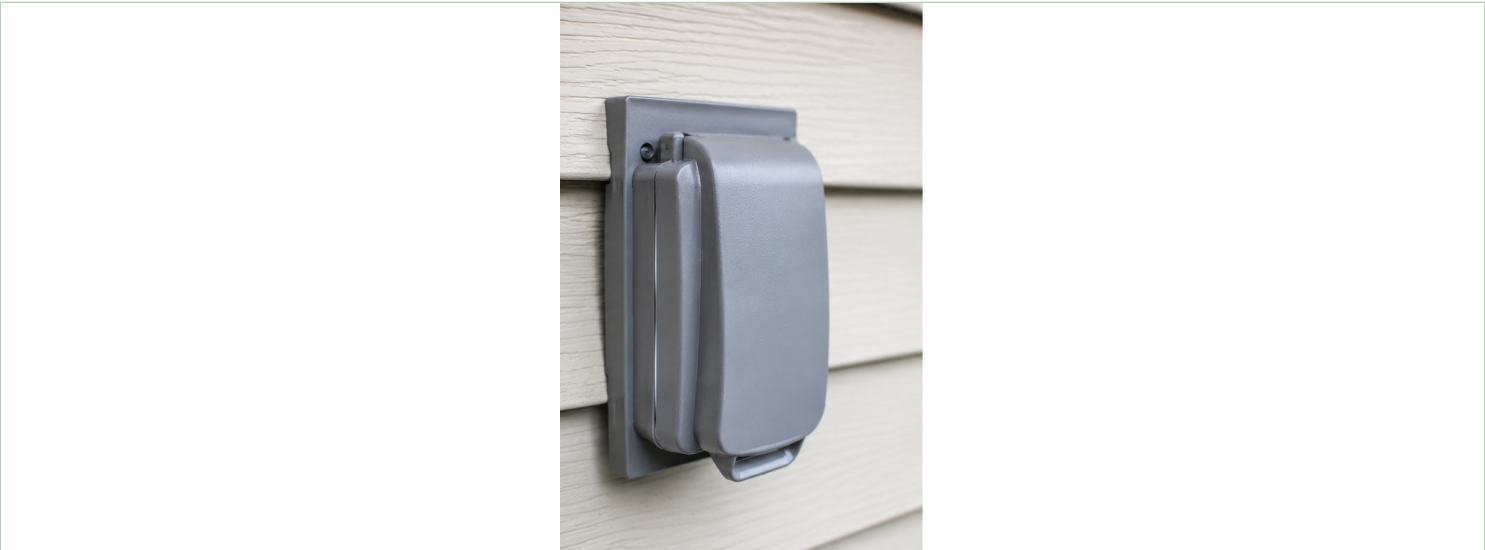
Outdoor receptacle covers must suit the location and use.
