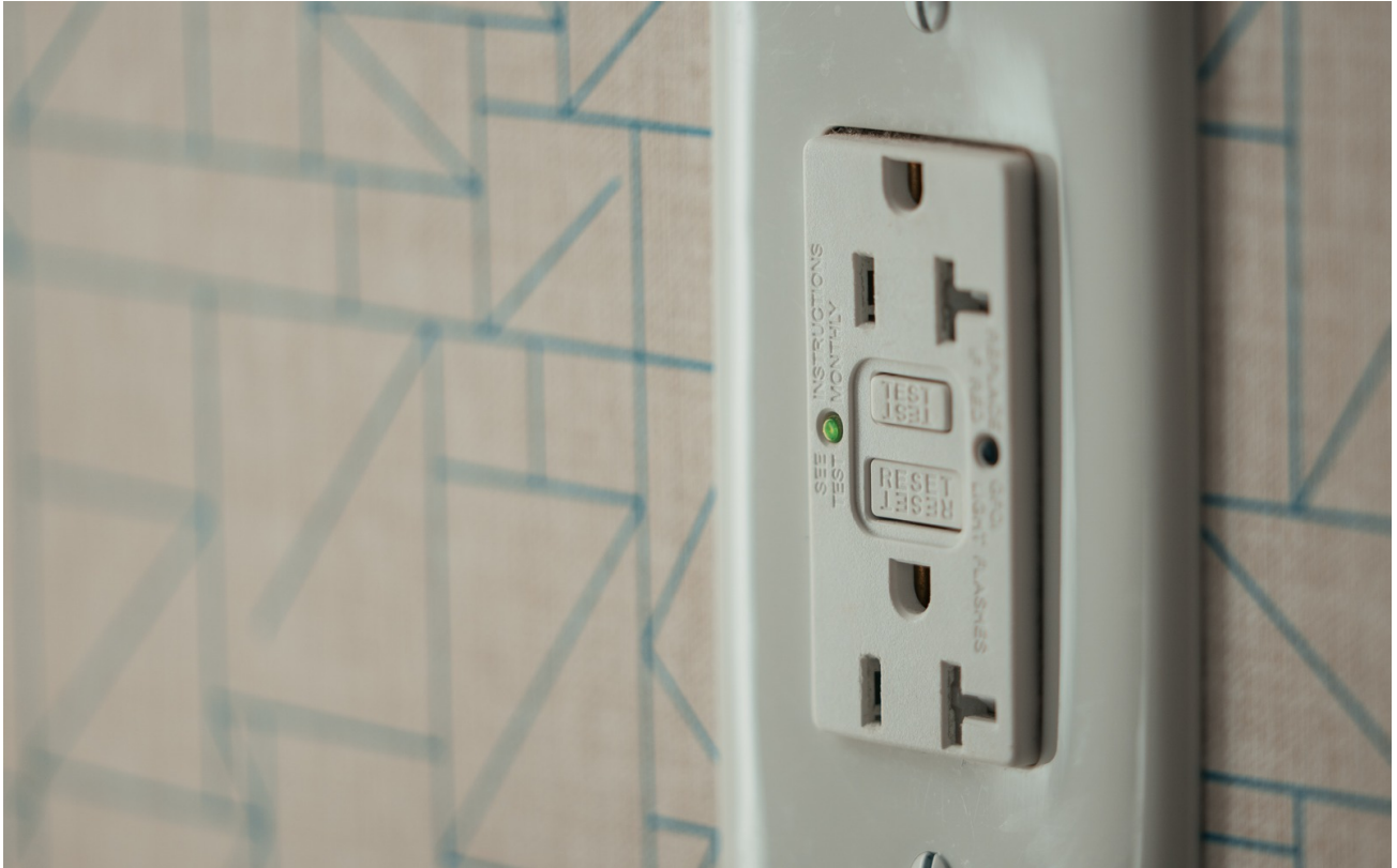
Figure 12-3 - Class A GFCI user interface concept
